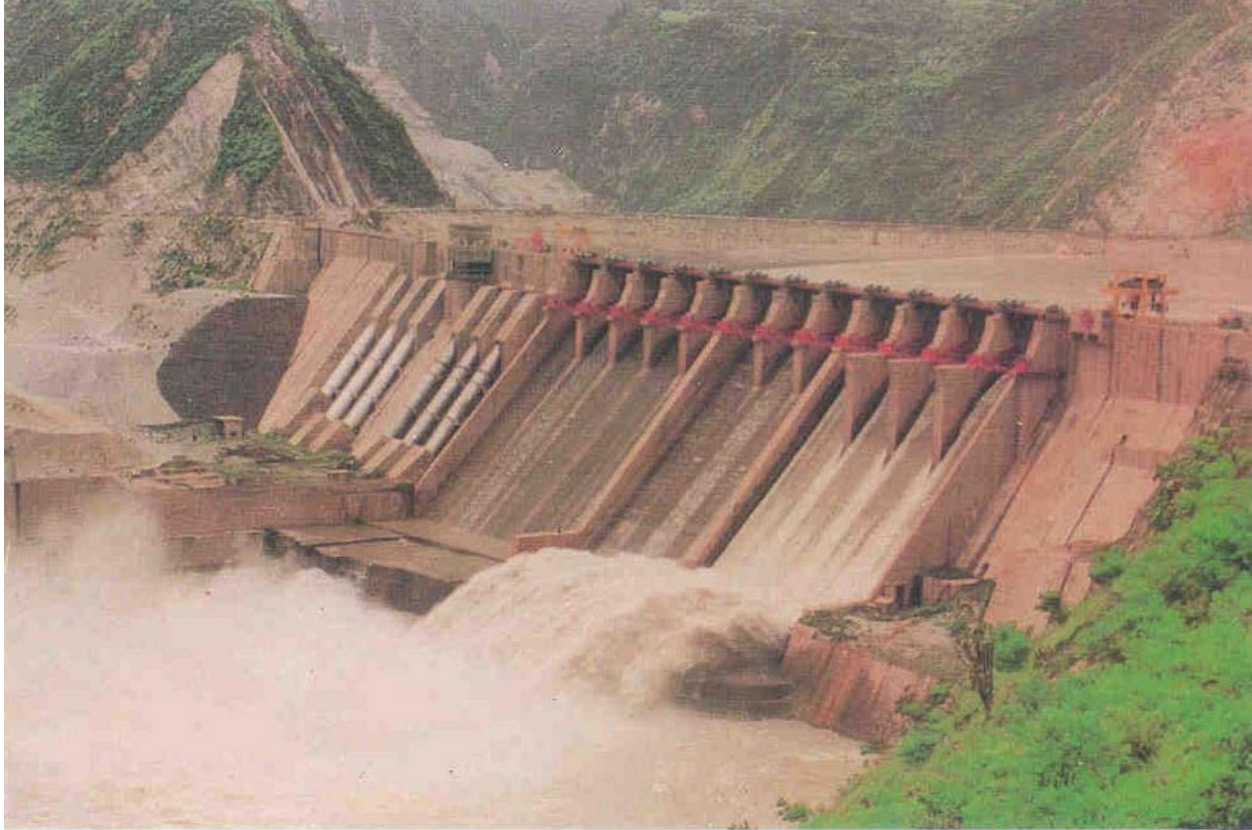
FIGURE 46. Salal project on river Chenab showing energy being dissipated by ski-jump bucket type energy dissipators
