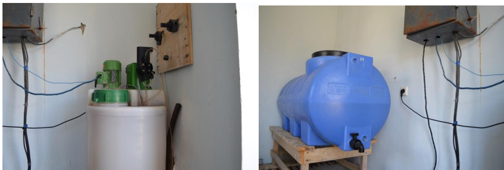
Figure 4-6: Sodium hypochlorite dosing station (the 2 nd pumping station PS-2 area)
