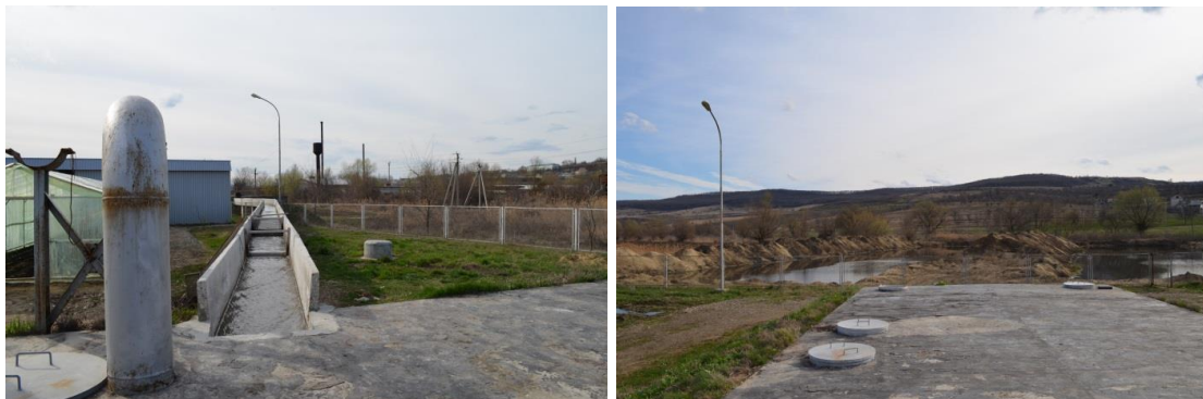
Figure 4-17: Wastewater treatment plant AquaClean MBBR: pumping / homogenisation / equalisation reservoir and biological ponds
