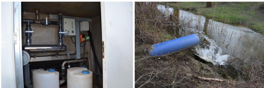
Figure 4-19: Wastewater treatment plant AquaClean MBBR: Ultraviolet lamps. Wastewater outflow into Bic River
