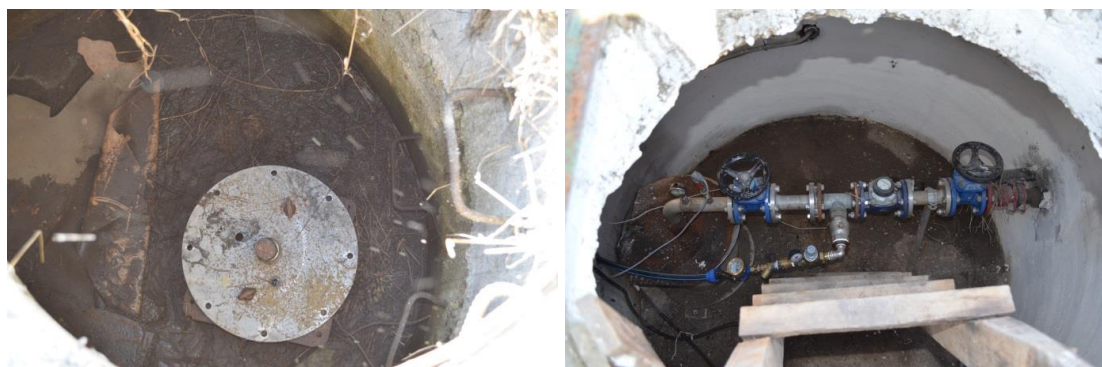
Figure 4-3: Deep well no. 4672 (9a). Water meter node
