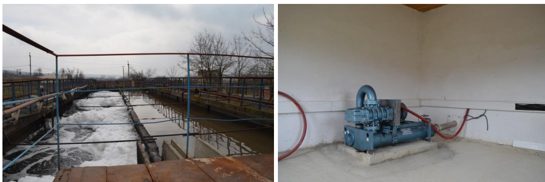
Figure 4-11: Wastewater Treatment Plant. Active sludge aeration tank. The blower
