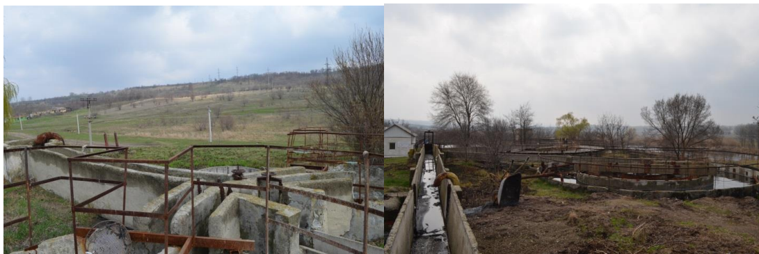
Figure 4-10: Wastewater treatment plant. Energy dissipater. Digester-settlers
