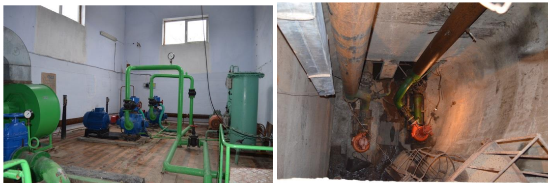
Figure 4-3: Raw water abstraction facilities. Pump group SEWATEC K200-4006-SEN 225M04. Pump group FA 15.84 DEMI-250/20
