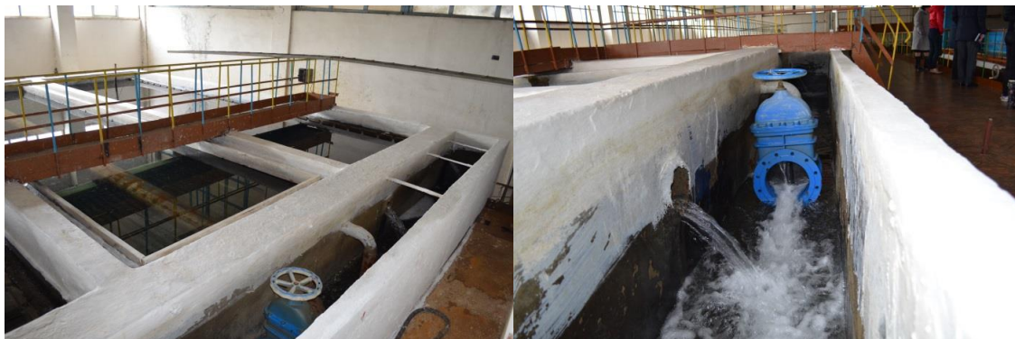
Figure 4-4: Water Treatment Plant. Horizontal longitudinal clarifiers
