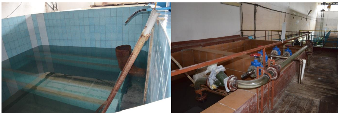
Figure 4-5: Water treatment plant. Open quick filter. Reagent building
