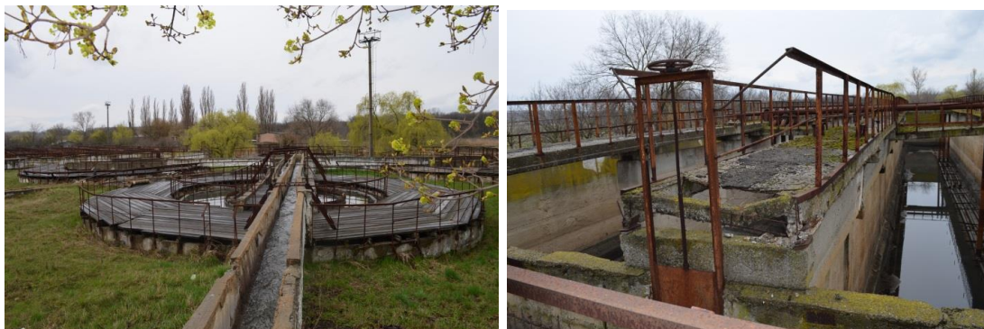
Figure 4-18: Wastewater treatment plant: Digester-settler. Active sludge aeration tank 9
