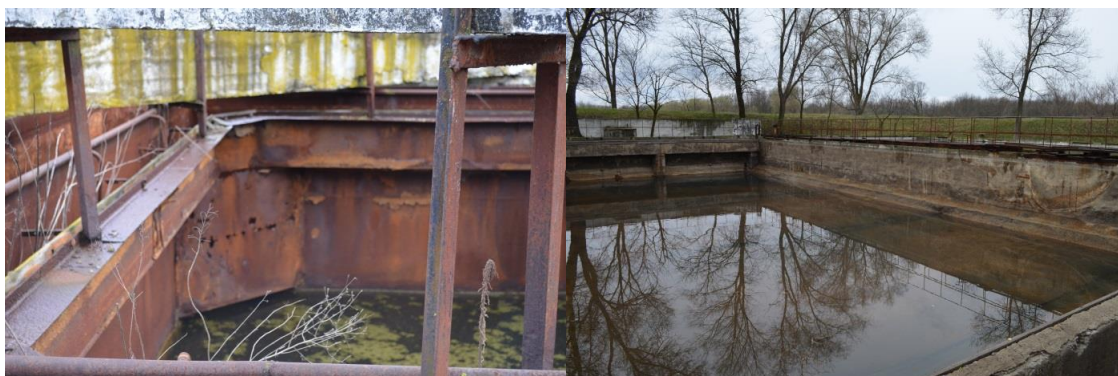
Figure 4-19: Wastewater treatment plant: Secondary settlers. Contact chamber
