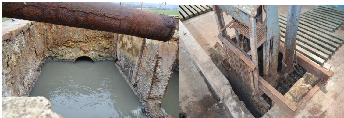
Figure 4-17: Wastewater treatment plant: Energy dissipater. Mechanical screens
