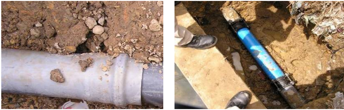
Figure 5 Typical repair of a leaking joint
