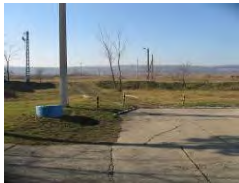
Figura 2.10-3: Front de captare
