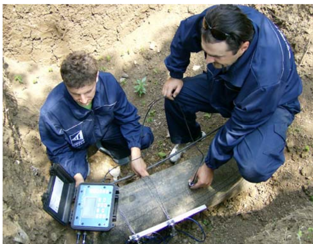
Figure 4. Flow measuring with Ultrasonic mobile flow meter
