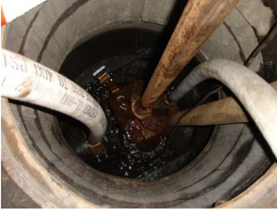
Figure 1: Bypass around a closed valve at DMA inlet
