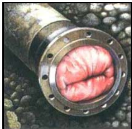
Figure 11 – 13: Pipe before rehabilitation / pipe with impregnated textile tube before heating / rehabilitated
