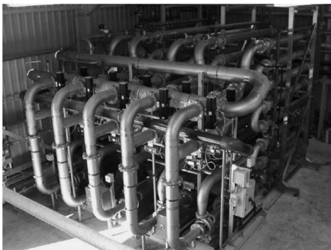
Fig. 12.7 Membrane modules in cross-flow mode. (a) Berghof tubular module and membranes. (b) Wehrle, MBR, ultrafiltration plant for the food industry.
