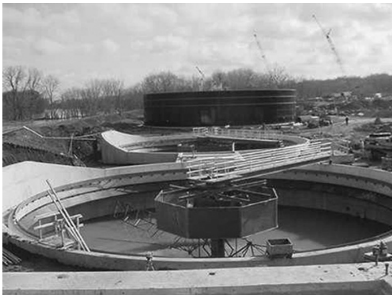
FIGURE 7.3 Circular clarifier under construction—Observed the center baffle that is used to direct the flow downward, under the baffle, before the flow flows outward to the launder ring (scum and floatable barrier) and the overflow weir around the periphery. Source: Greeley and Hansen-Lafayette, Ind.
