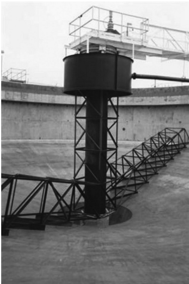
FIGURE 7.4 Innards of a sludge thickener. Note steeply sloping sides and mechanical rake which promotes sludge compaction & collection in the center well. Other manufacturers will have tanks with steeper sides and vertical poles (rakes) on the collector mechanism to promote thickening. Photo courtesy Wes-Tech Engineering Salt Lake City, UT.
