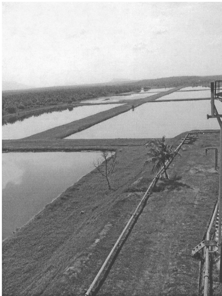
Figure 4.4 A series of ponds for POME treatment occupying a large land area. (Courtesy of Felda Palm Industries.)
