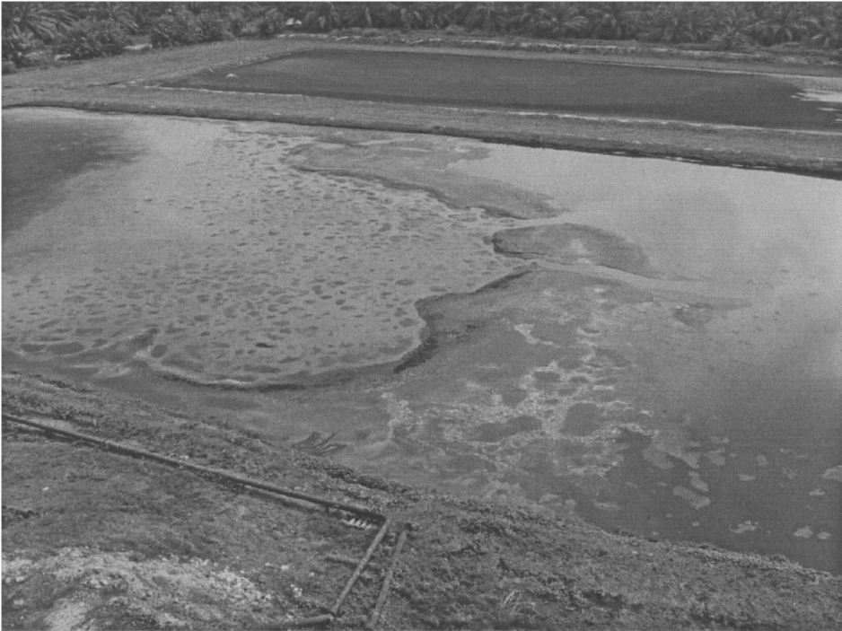
Figure 4.6 Formation of islets of sludge in the middle of the pond. (Courtesy of Felda Palm Industries.)
