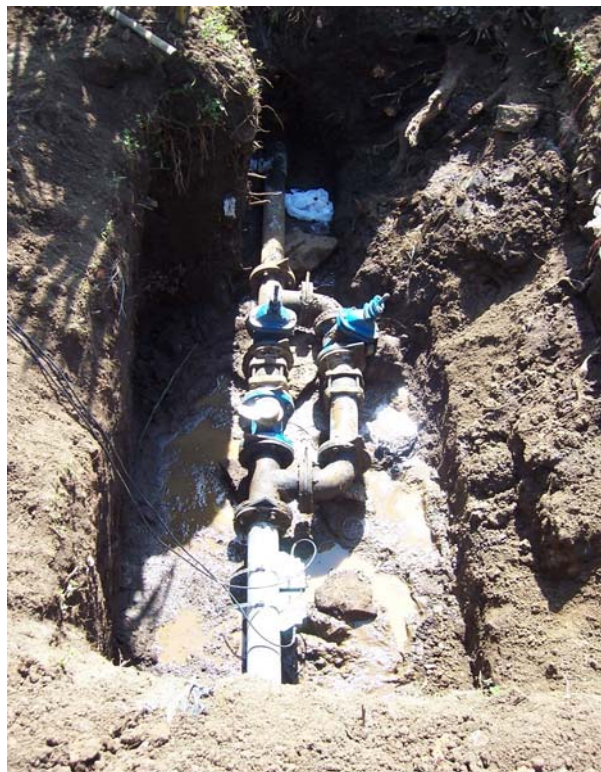
Figure 3 A Sub-Standard DMA Measurement Chamber
