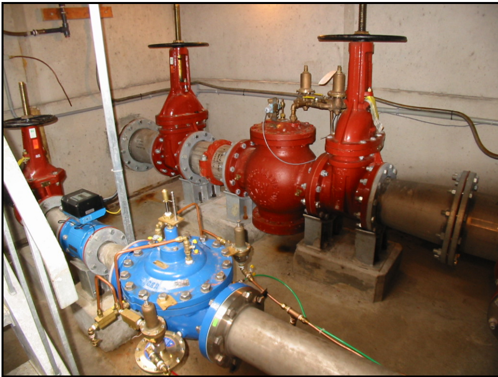
Figure 2 Standard HRWC supply chamber configuration
